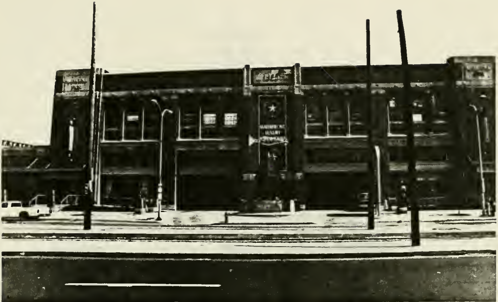
PLATE 9 Pier 5, west facade
